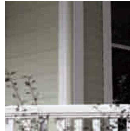
Trimworks Three-piece beaded corner post.
